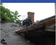
just about complete on the library roof resto- Browsing Room. ration project. Damaged slates have been replaced, usable reused, flashing
